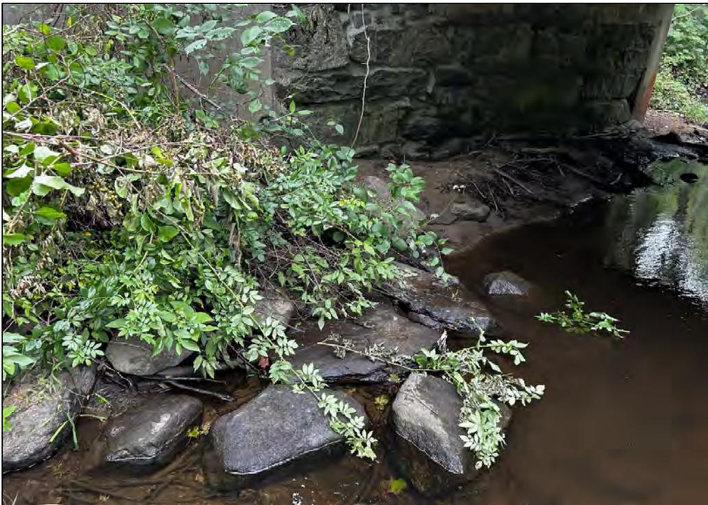
Photo 4. Eastern abutment of Bridge 04730 showing accumulated sediment along the northern side preventing OHW painting.
