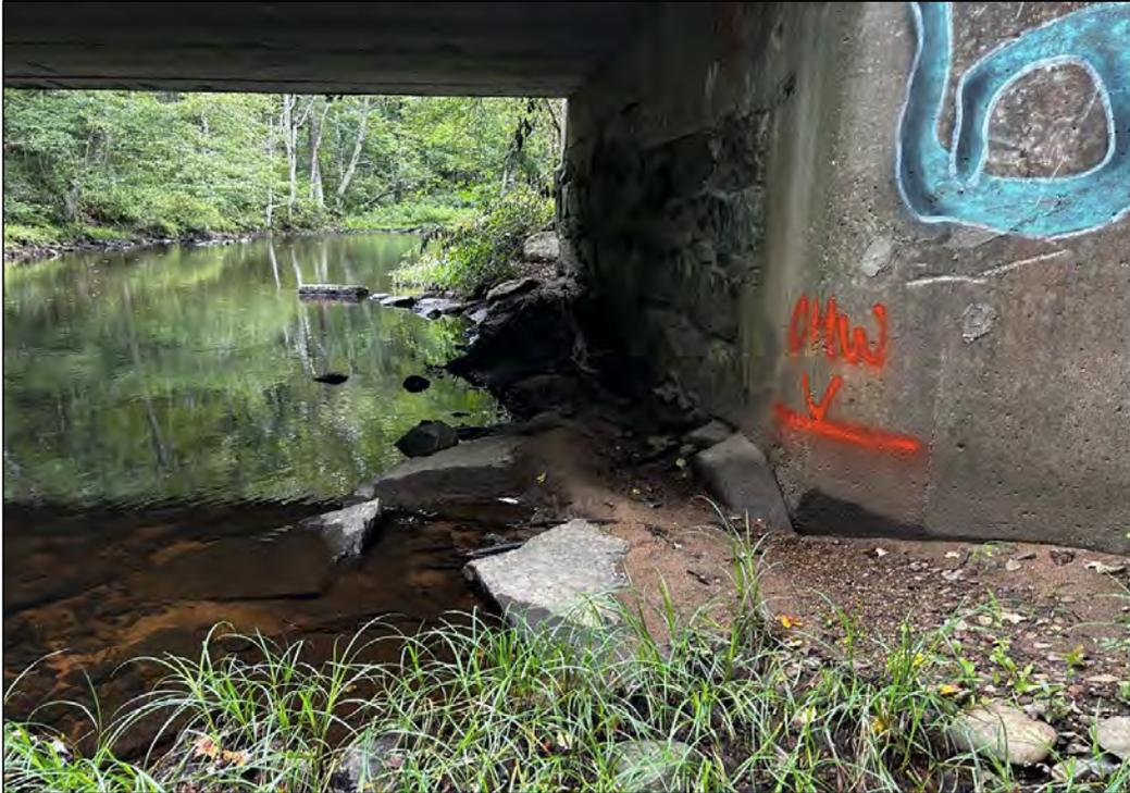
Photo 3. OHW indicated on the eastern abutment of Bridge 04730. Photo facing north.
