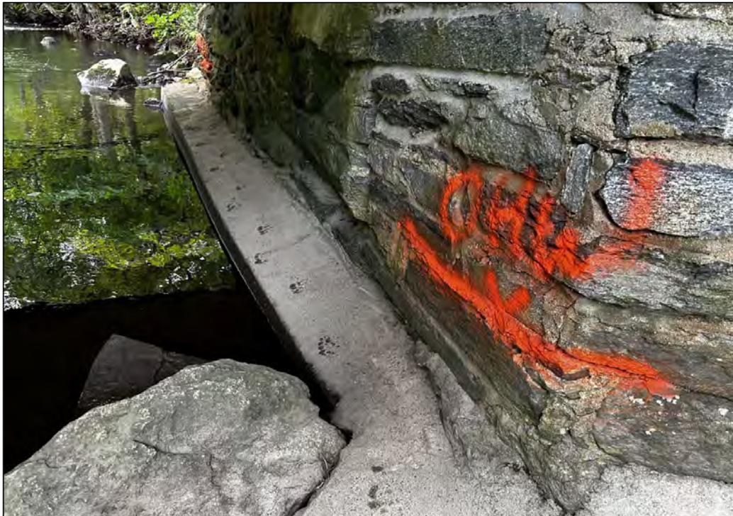
Photo 6. OHW painted on the western abutment of Bridge 04730. Photo facing south.
